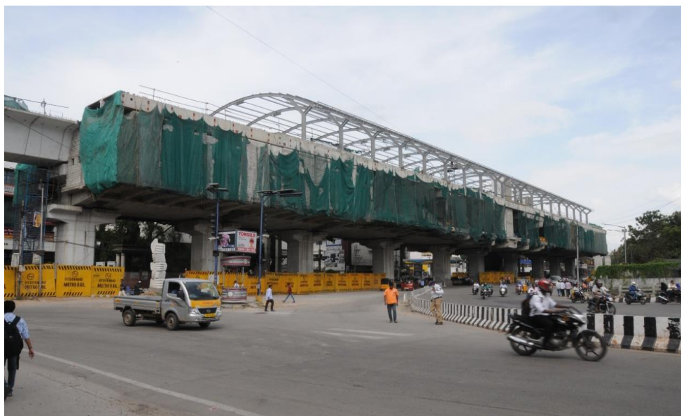
Metro Station Construction-Roofing Stage
