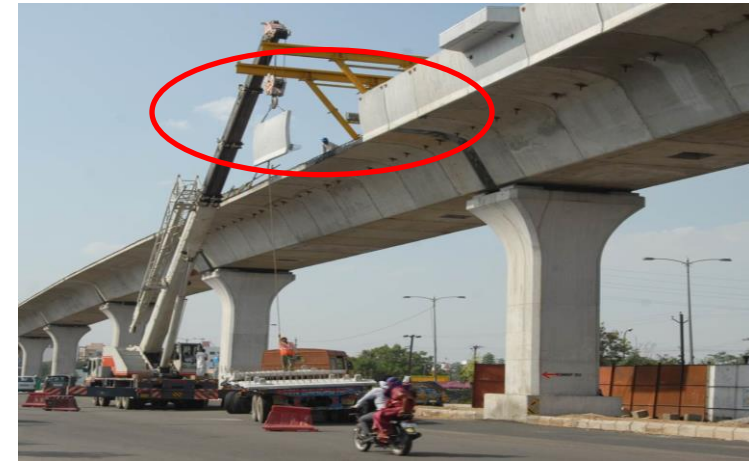
Erecting Parapet Wall on the Viaduct
