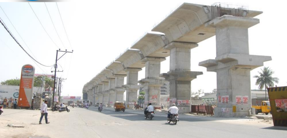
Metro Station Construction-Pier & Segment Stage
