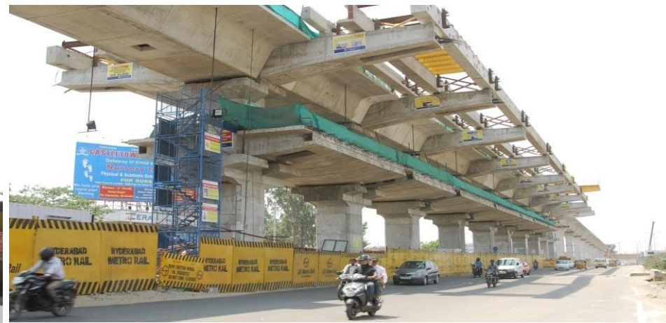
Metro Station Construction-Spine & Wings Stage
